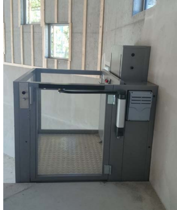
Upper gate with automatic door opener
